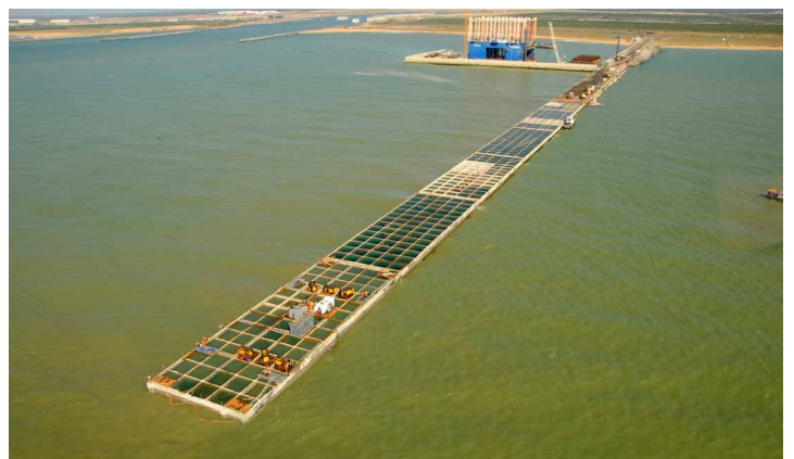
▲ Açú Port (São João da Barra, Brazil): 2 mixed jetties. Caissons and rockfill. Length: 4.895 km.
