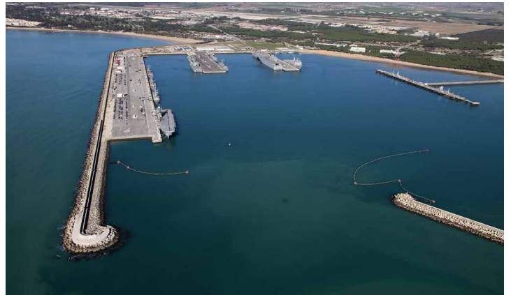
▲ Rota Naval Base (Cadiz, Spain): Caissons and rockfill. Concrete: 61,166 m 3 . Steel: 4,982 MT.
