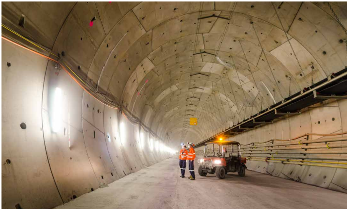
▲ Legacy Way (Australia): Tunnels: 2 x 4.26 km. Contract: AUD 1.5 billion.
